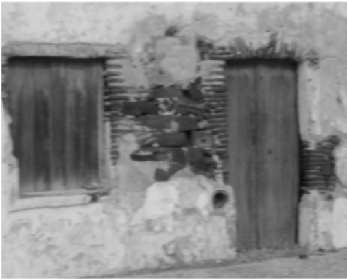
Figure 2. Trim reinforcement with lambaz brick (Credits: CI-ESG, 2013).
