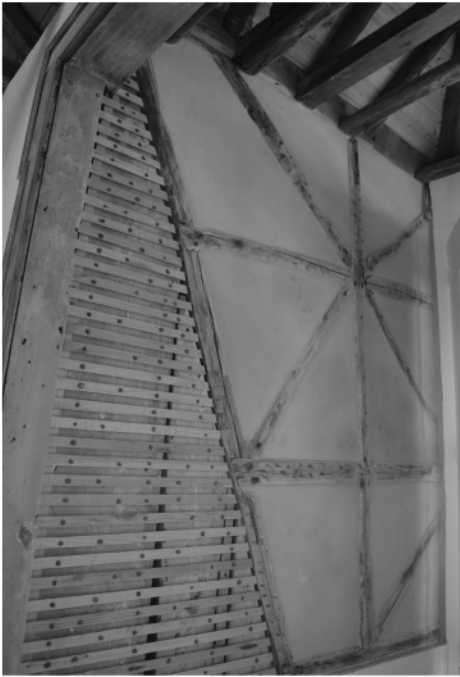
Figure 6. “Gaioleiro” system in Vila Real de Santo Antonio (credits: CI-ESG, 2015).
