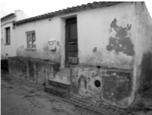
Figure 3. Rammed-earth building with reinforced plinth course, Bensafirim (Credits: CI-ESG, 2013).
