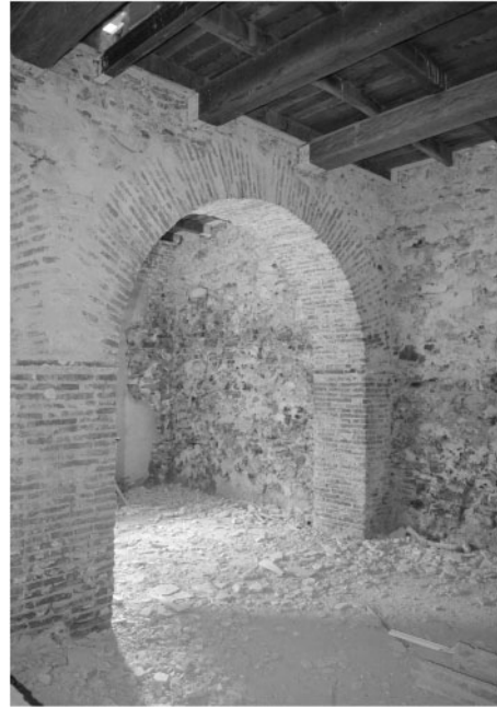
Figure 7. Covering system sustained by arches in Vila Real de Santo António (credits: CI-ESG, 2015).
